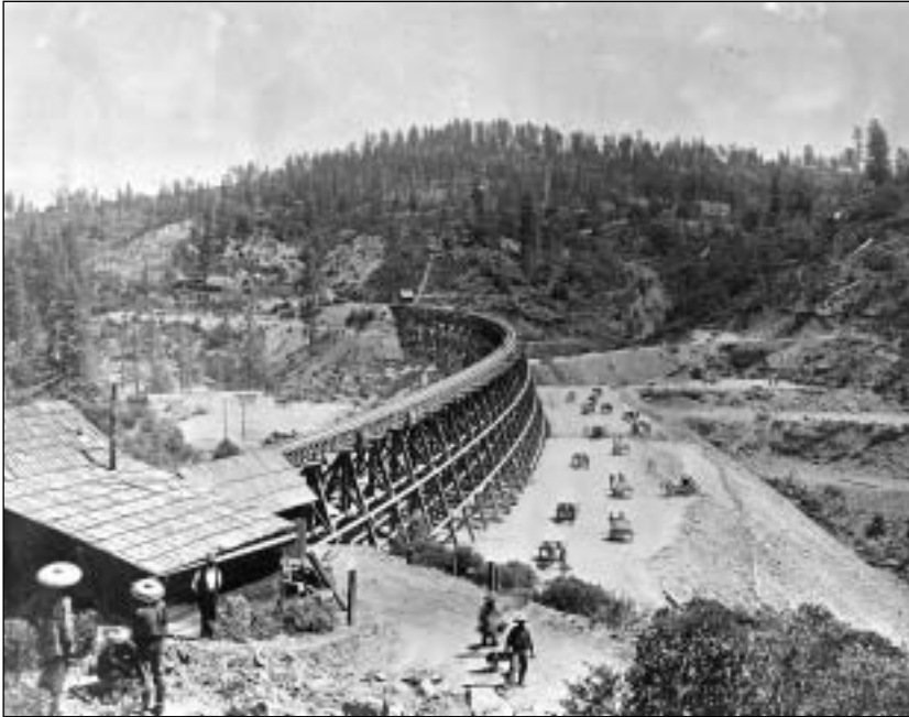
49. Chinese laborers with hand tools and carts working on the Secrettown trestle in the Sierra Nevada in 1866. Union Pacific Collection .
