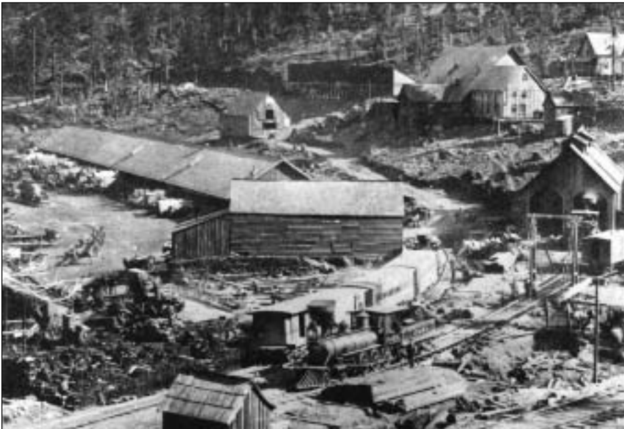
50. Railroad construction in Cisco, 1866. Union Pacific Collection .
