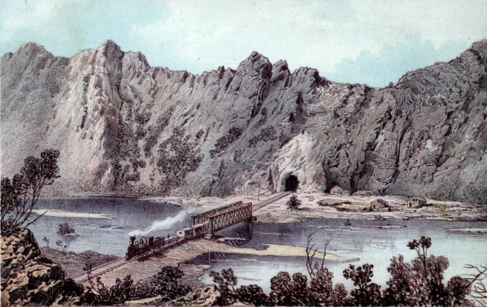
TUNNEL AT WEBER CANYON.
